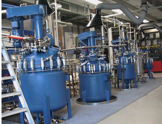
Fig. 7.3. Fermentation plant, University of Regensburg. Partial view, showing two 300 l fermentors and one 130 l fermentor for cultivation of HT.
